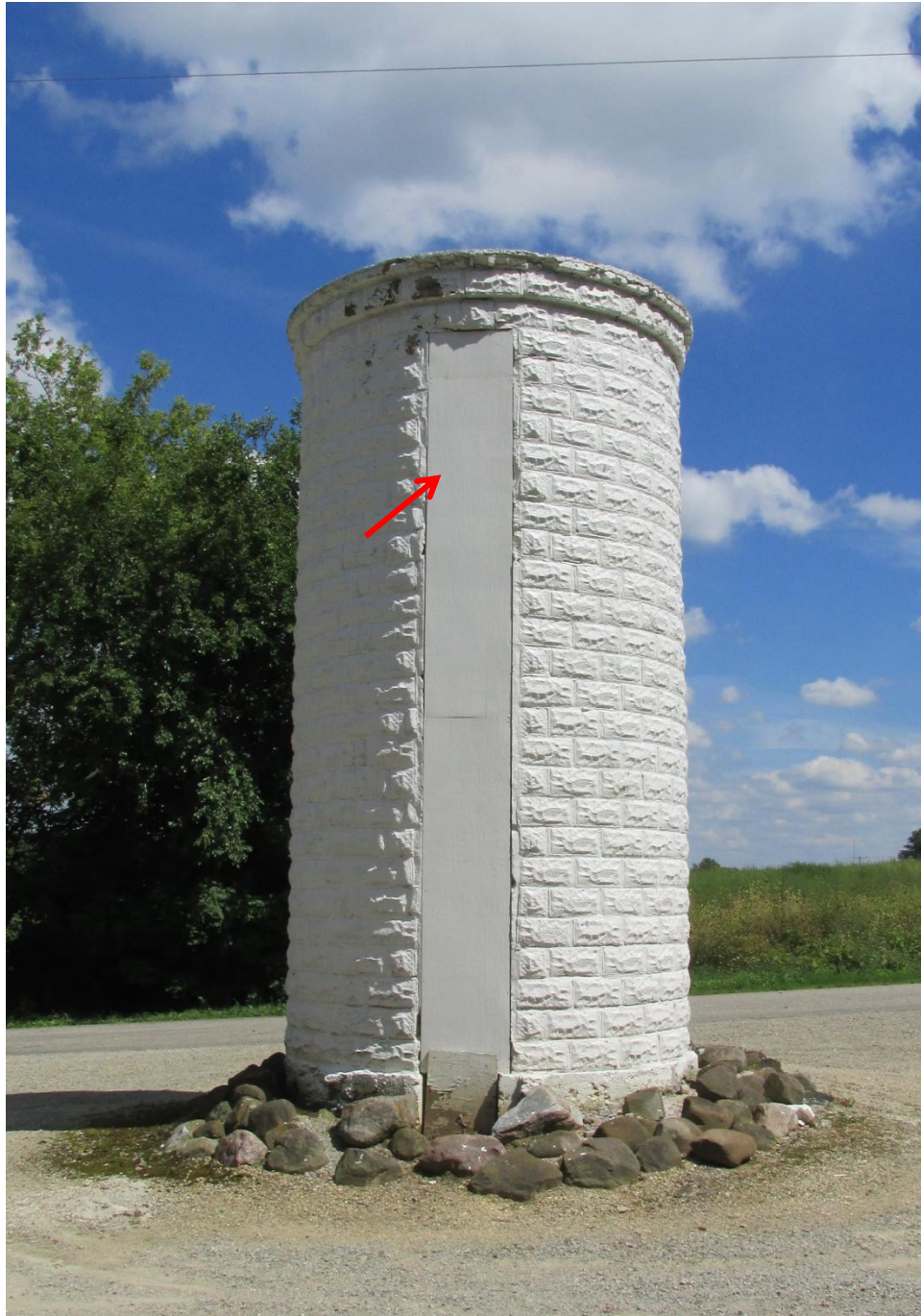
Photo 1: West Elevation of Silo (Arrow Points to Plywood Cover)
