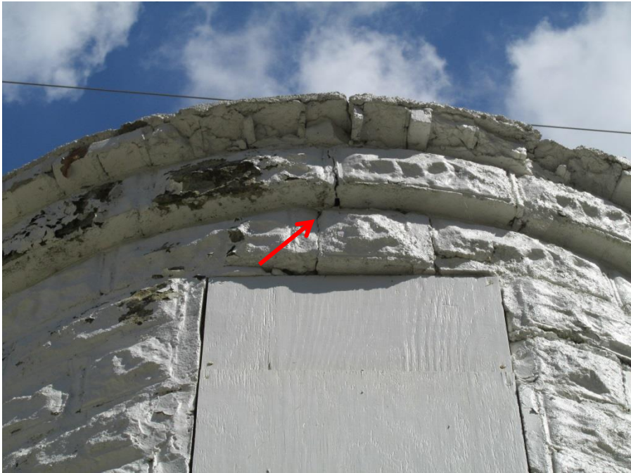
Photo 5: Step Crack at West Elevation
