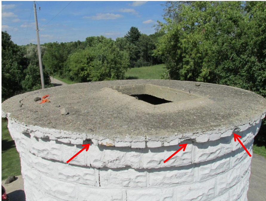
Photo 2: Silo Cap w/ Rectangular Opening (Arrow Points to Missing Brick)
